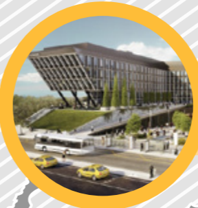
Office complex in MOSCOW
